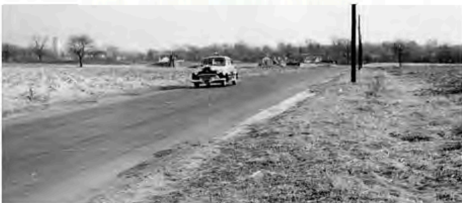
Warwick Road, cutting through the Stafford Farm, looking toward Laurel Springs and Stone Road, 1953. Future site of Stratford Estates.
