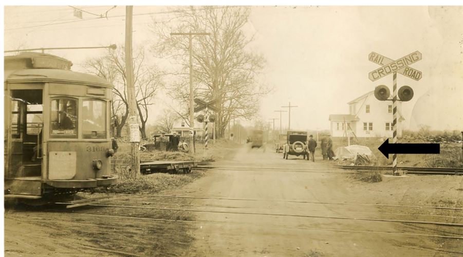
In 1922, a train hit a car at Laurel Road and Atlantic Ave. The wreckage can be seen covered, behind the signal. The Camden/Clementon Trolley is seen approaching Laurel Rd.
