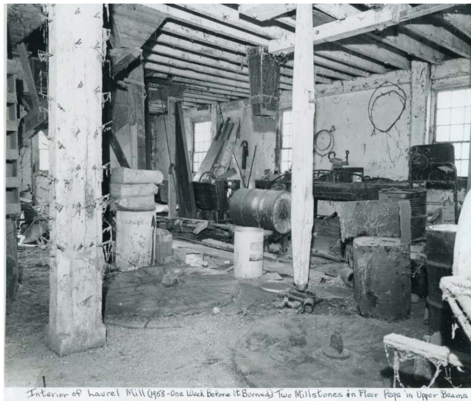
Interior of Laurel Mill in 1958, one week before it burned down. Two Millstones sit on the floor while one of the grinding pegs hangs from the beams
